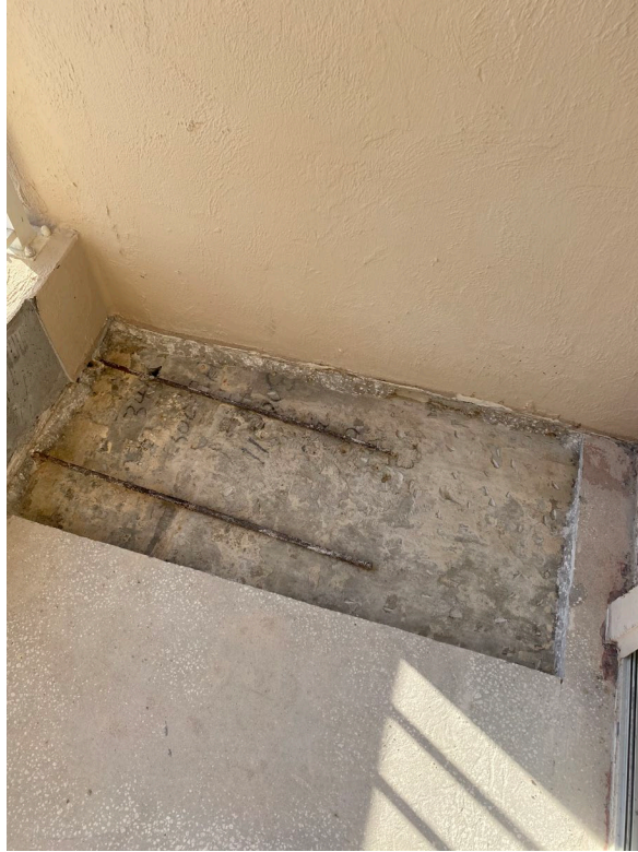
Picture 1: Typical concrete repair
