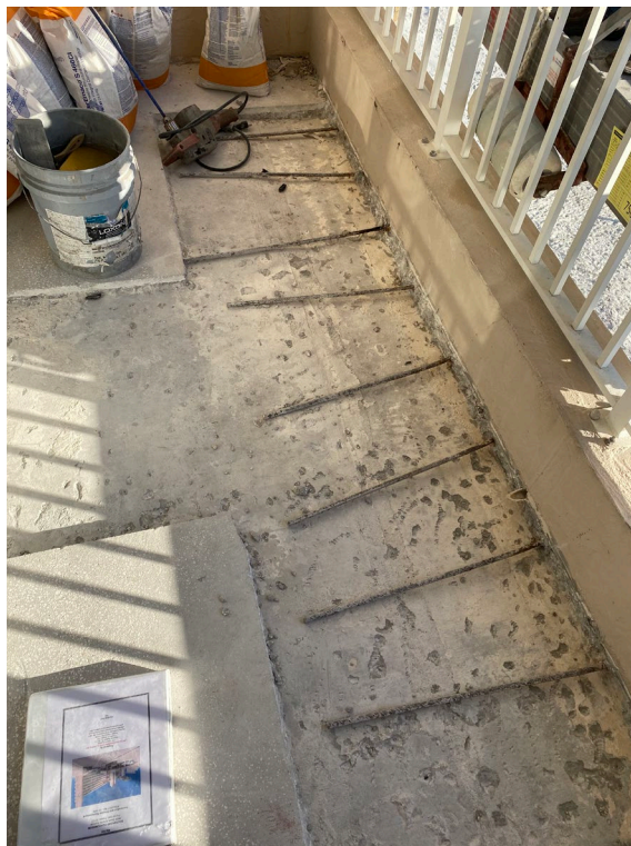
Picture 3: Typical concrete repair
